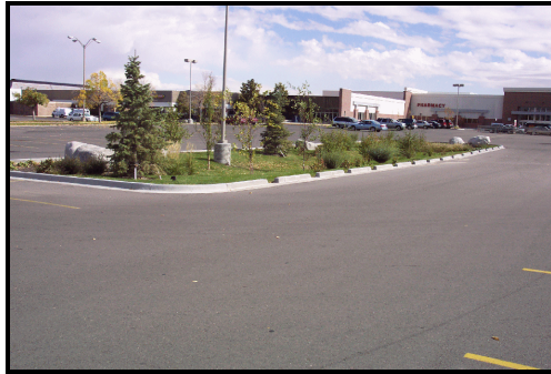
Figure VII-3. Examples of Curb Breaks for Stormwater Runoff
