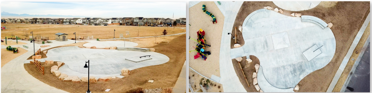
Turnberry Skate Park, completed in 2021, enhanced the Turnberry Park amenities with beginner skate elements for youth and residents.
