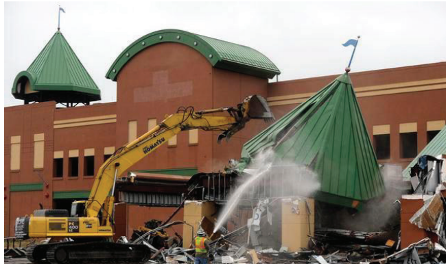
Old clubhouse being demolished.
