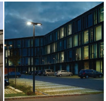
Tall pole top fixtures in vehicular areas.
