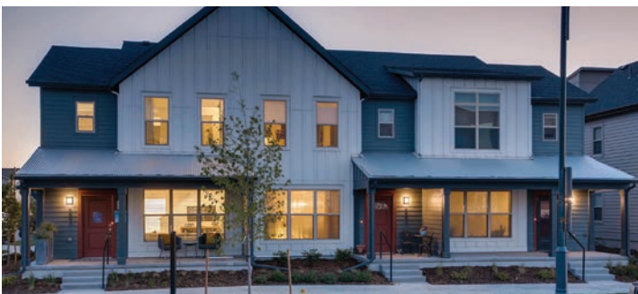
No garage facing street - duplex.
