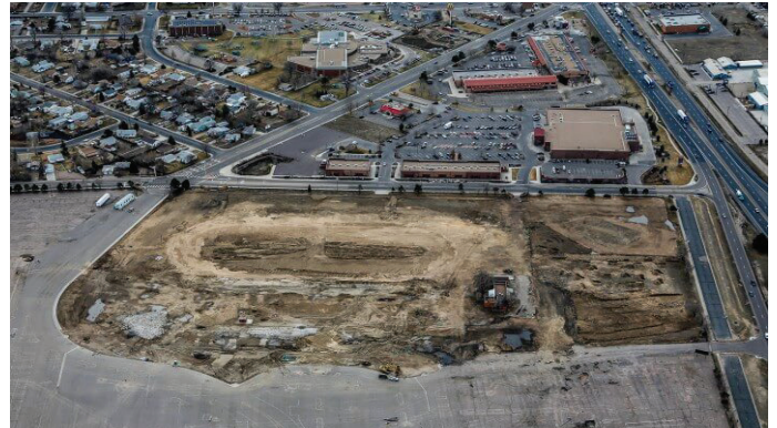
The site after demolition.
