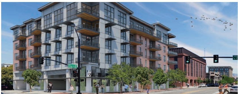
Awnings, balconies, & overhangs animating a building facade.
