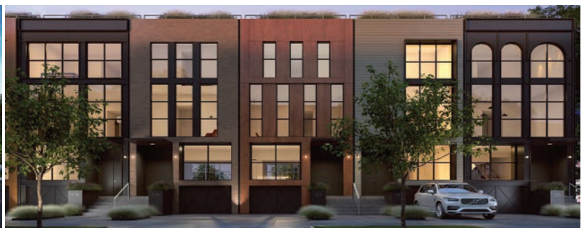
Building parallel to a street with direct access to sidewalk.
