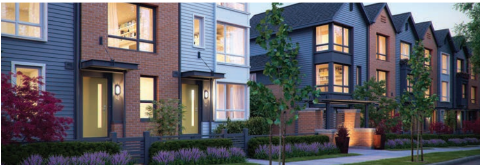
Amenities like benches and landscaping create a pedestrian friendly environment.
