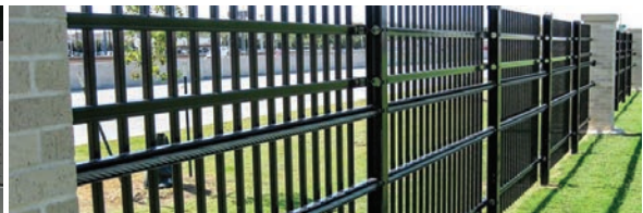
Open slat fence with visual permeability.
