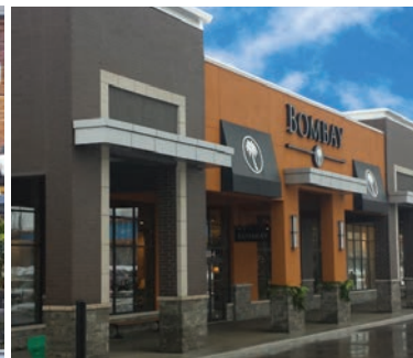
Effective use of stucco & brick.
