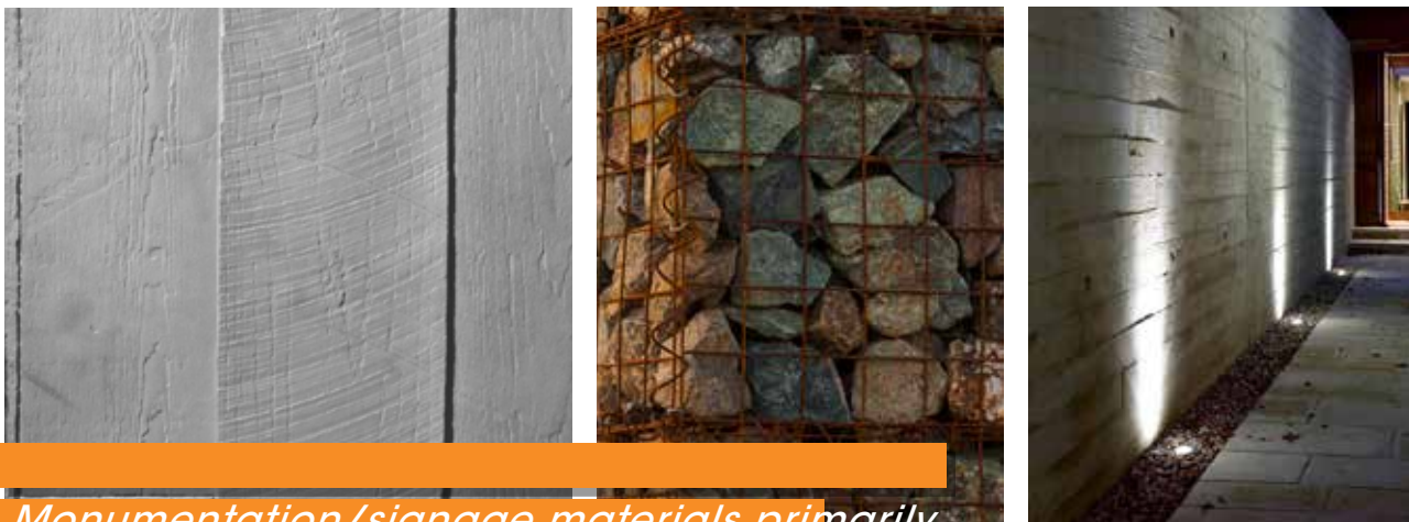
Monumentation/signage materials primarily include board formed concrete, stone,
