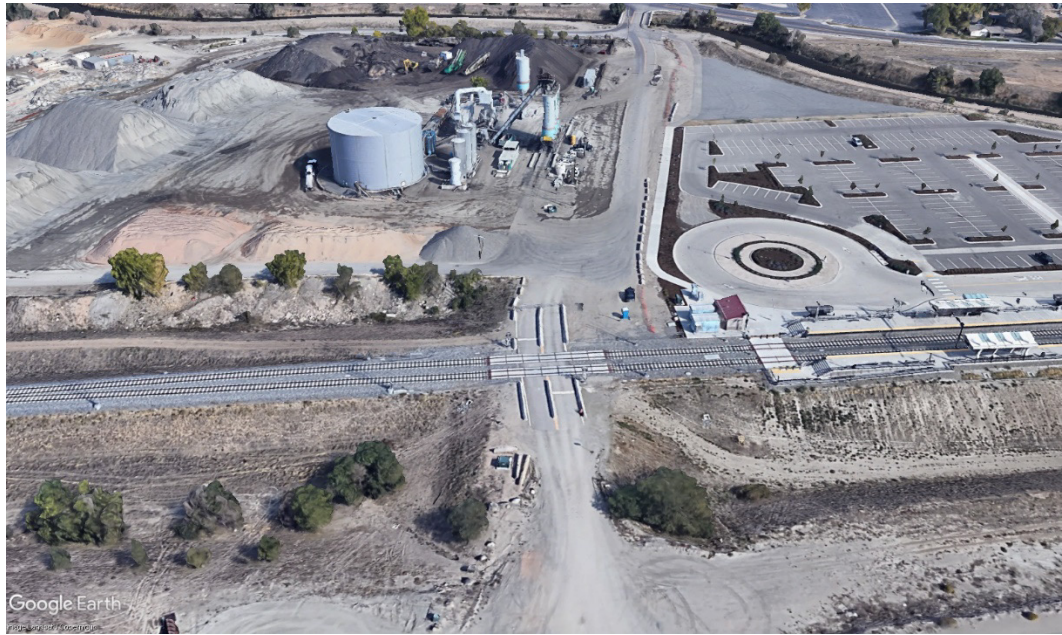
Figure 3. Inadequate emergency vehicle access
