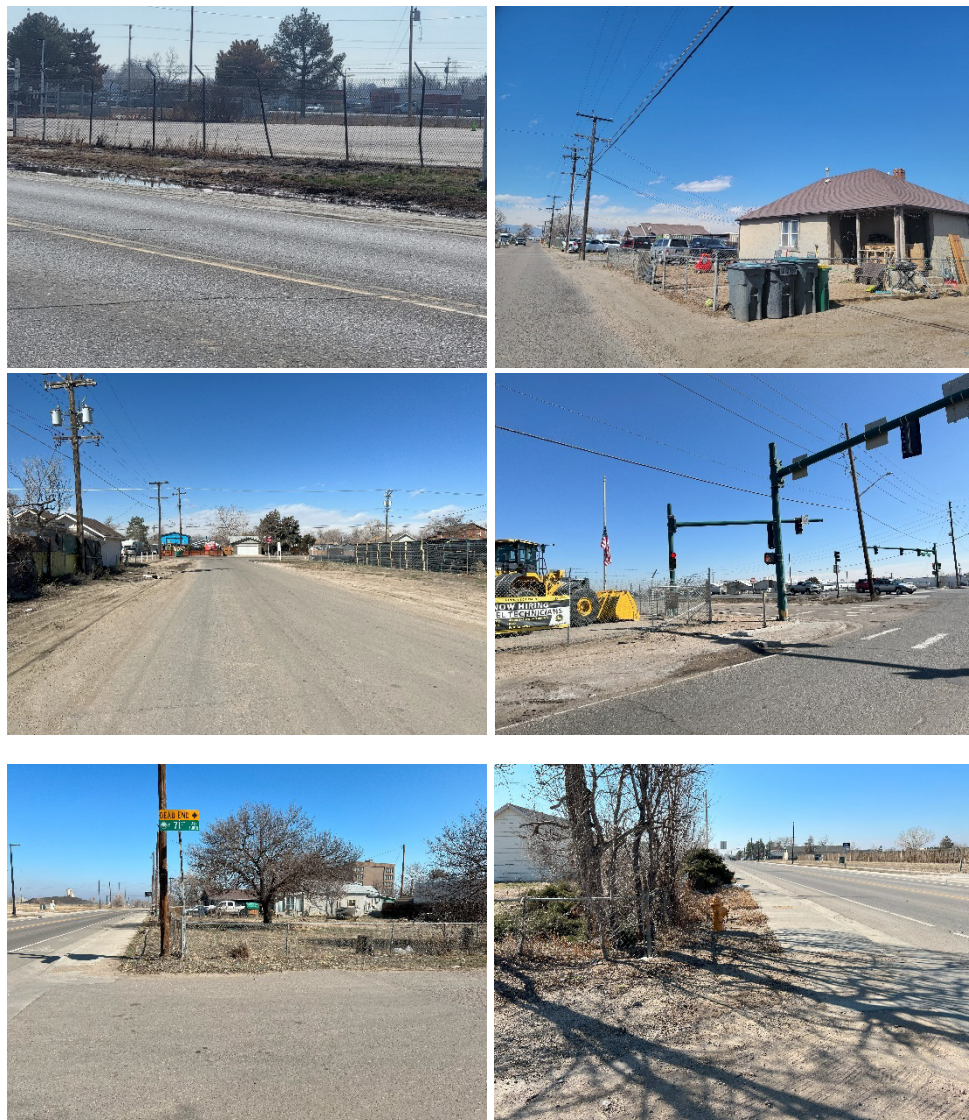
Figure 4. Poor provisions or unsafe conditions for pedestrians
