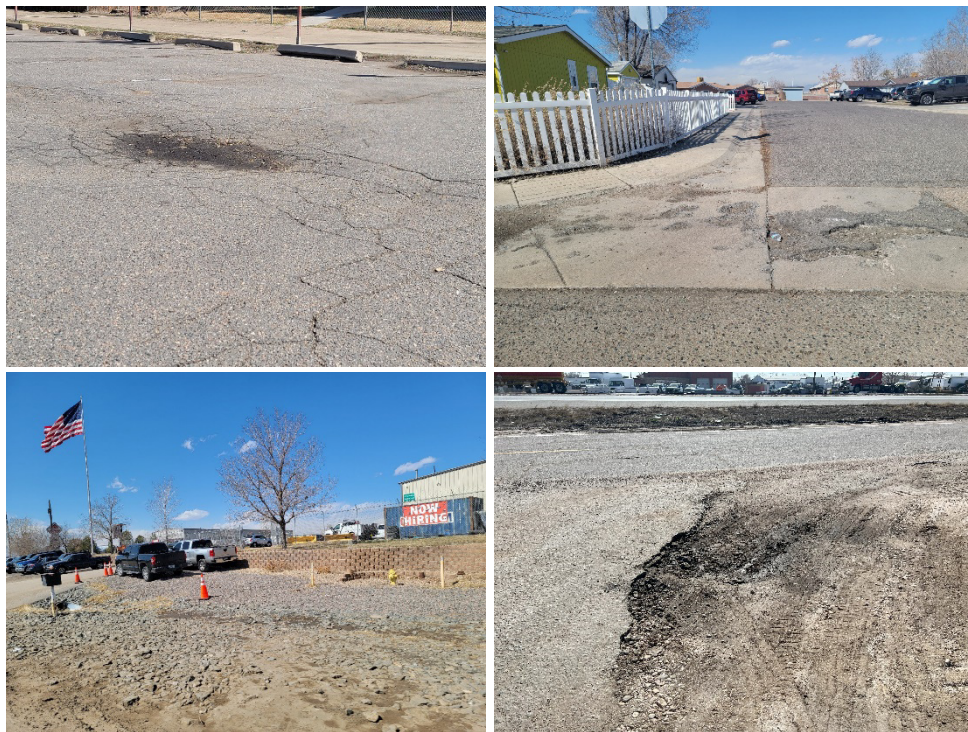
Figure 2. Poor provisions or unsafe conditions for vehicular traffic
