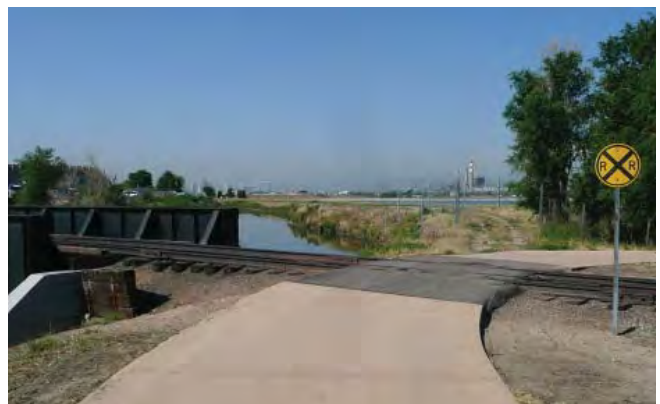
The O'Brian Canal trail should become a community amenity and new connection to the Sand Creek Greenway
