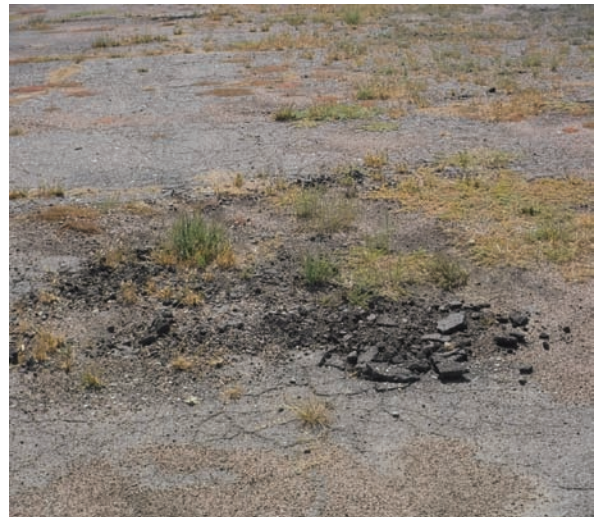
Deteriorated Paving
