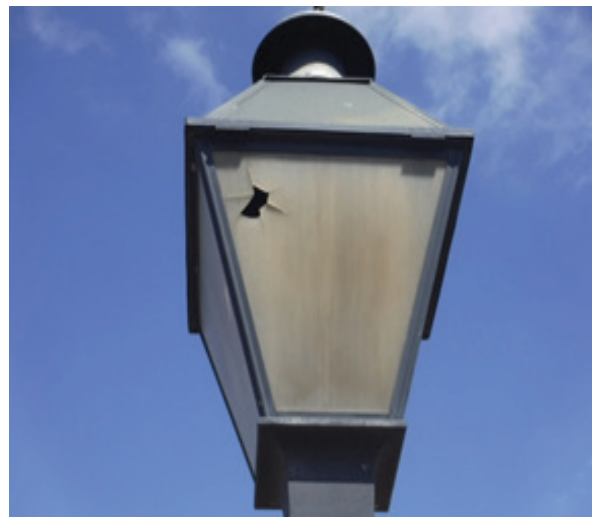
Deteriorated Light Structure
