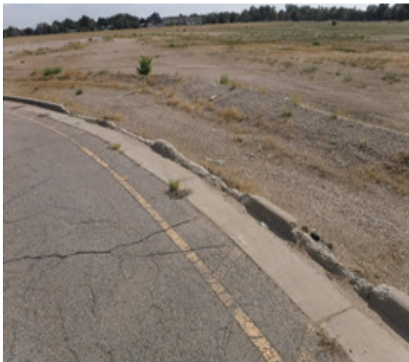
Deteriorated Curb
