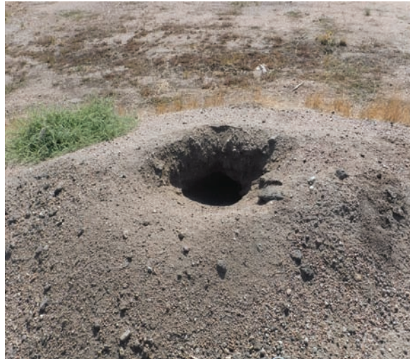
Evidence of Rodent Infestation
