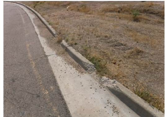
Deteriorated Curb/Sidewalk
