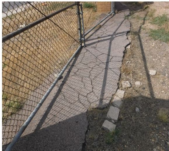
Blocked/Poorly Maintained Emergency Access
