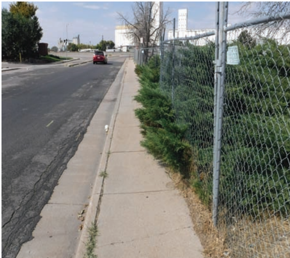
Pedestrian Barrier Resulting in Vehicle Conflict
