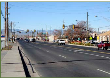
72nd Avenue is a wide minor arterial
