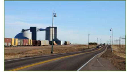
SH 2 will need to be widened to 4 lanes
