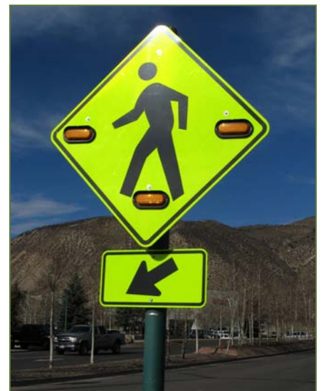
Pedestrian-actuated flashing beacon
