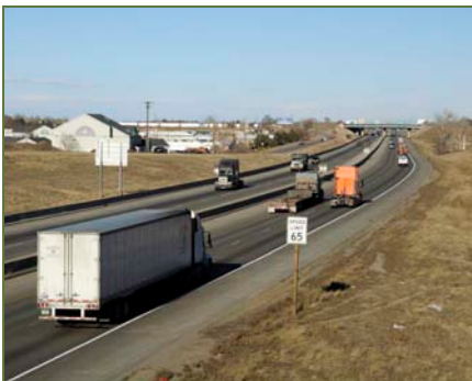
I-76 north of Dahlia Street
