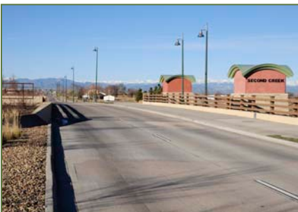
This bridge on 104th Avenue over Second Creek was recently constructed
